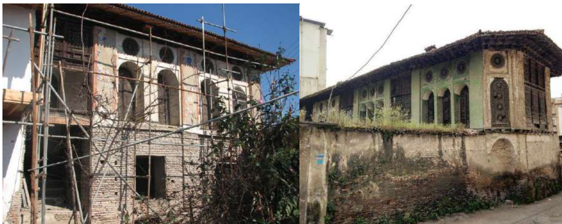
Figure 2. South view of Qureshi House
